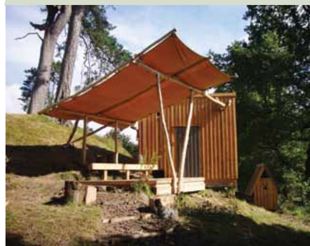
This example of a simple, off grid hut was designed by Alastair Baird. Compost toilet visible in the background. Photo: Falkland Centre for Stewardship.
