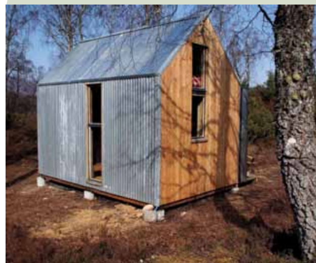
Located within the Cairngorms National Park, Inshriach Bothy was designed by architect Iain MacLeod and artist Bobby Niven. Photo: The Bothy Project.
