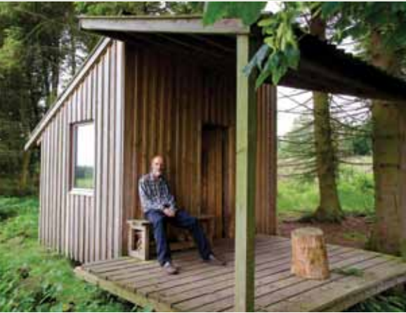
Ninian Stuart at his hut near Falkland. This design has a 6m 2 deck under a lean-to roof integrated with a 16m 2 hut. Photo: Alastair Stephen.
