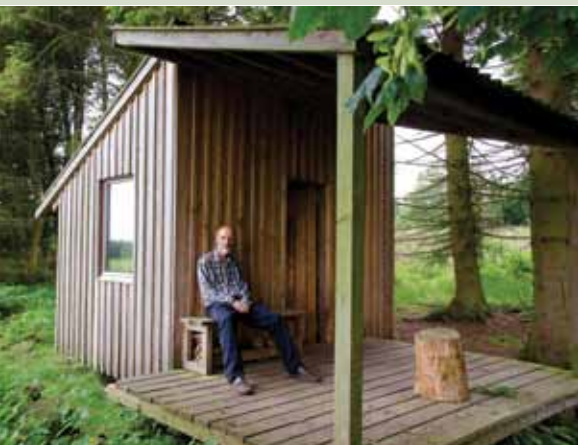
Ninian Stuart at his hut near Falkland. This design has an 8m 2 deck under a lean-to roof integrated with an 8m 2 hut. Photo: Alastair Stephen.
